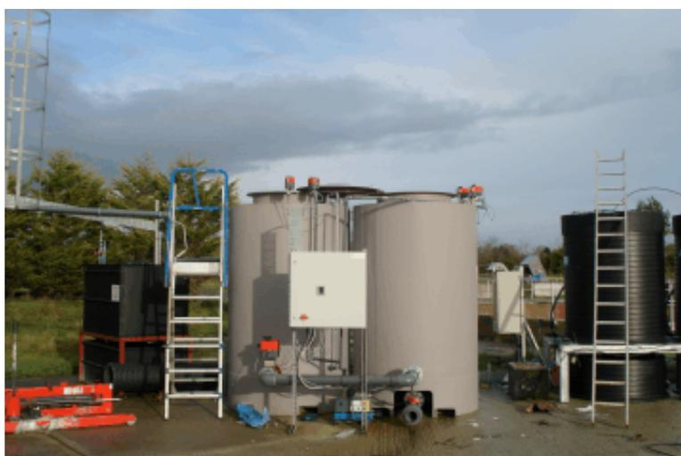
Figure 6.6. Pilot-scale air-suction flow biofilm reactor units at the Water Research Facility.
