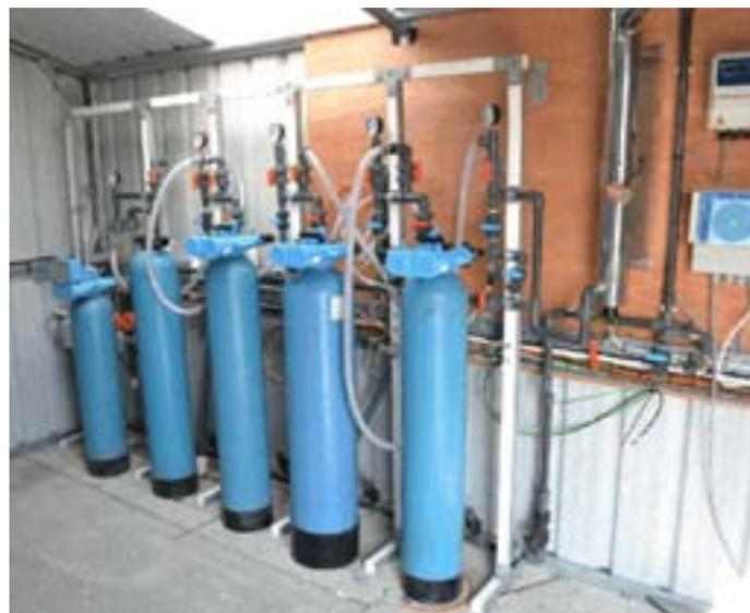
Figure 5.4. Picture of the tertiary treatment system installed at the Water Research Facility.
